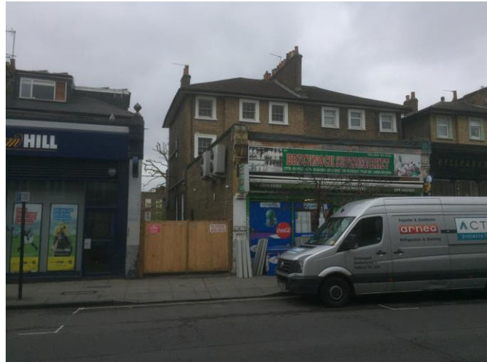
View towards front elevation of 43 Brecknock Road
