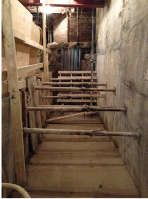
Figure 4 Examples of completed walls and back propping to central soil mass
