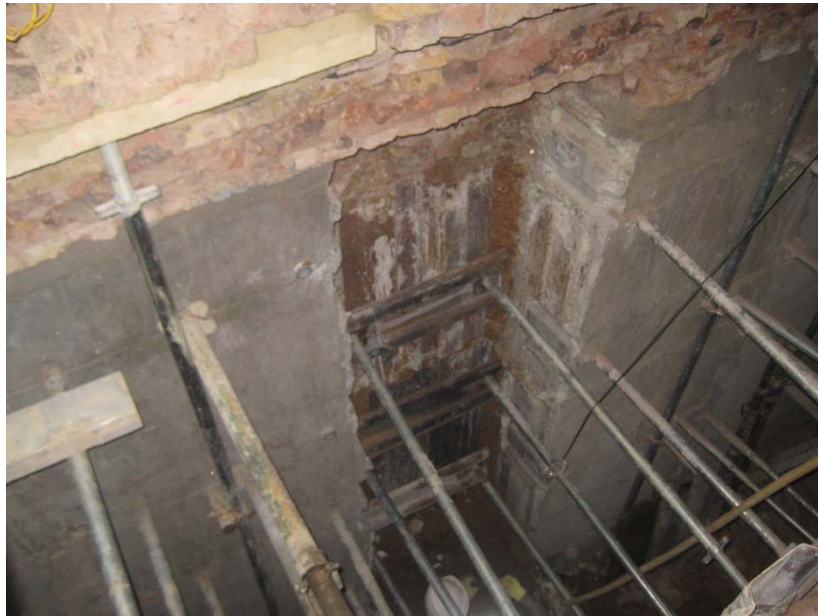
Figure 5 Example of trench sheet back propping
