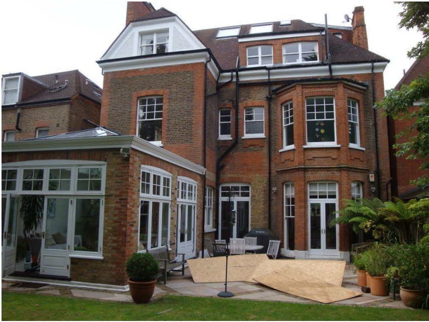
Rear Elevation . general view
