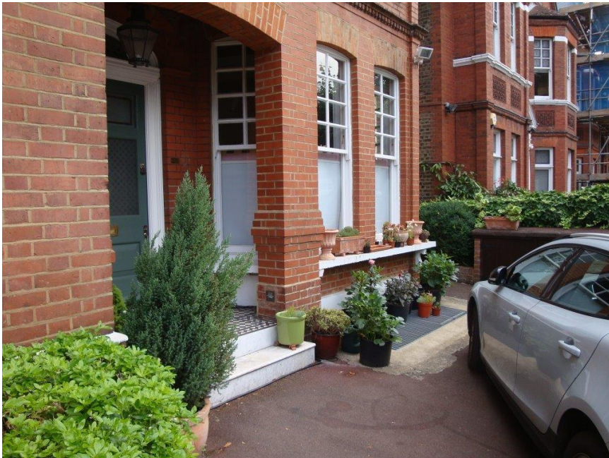
View to existing lightwell
