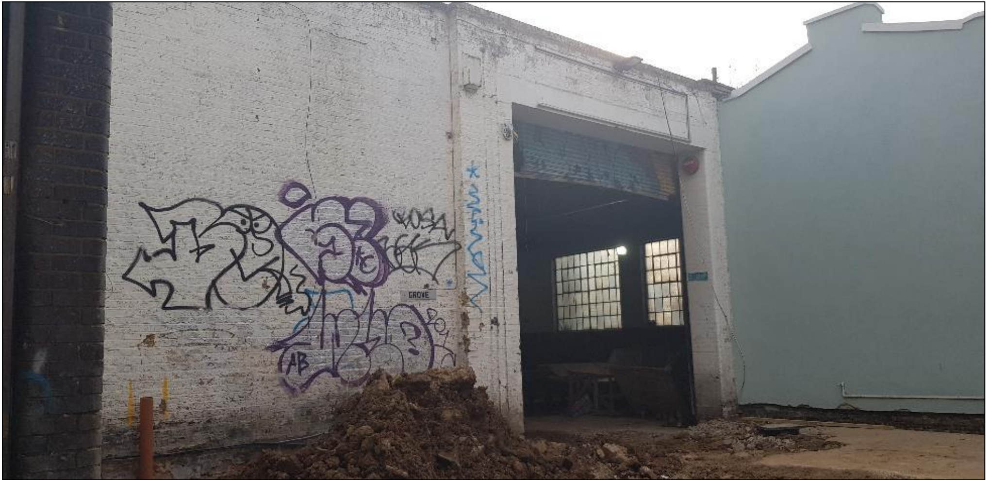
Photo 5: The western elevation of the subsection of B1.
