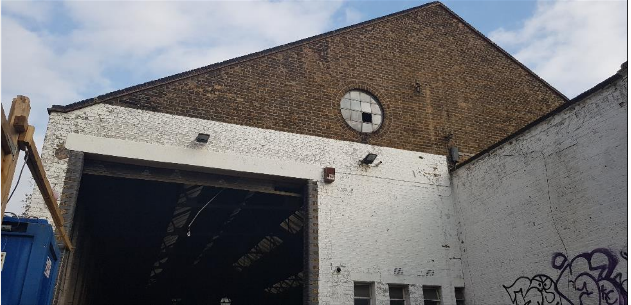
Photo 4: Southern elevation of the main section of B1.
