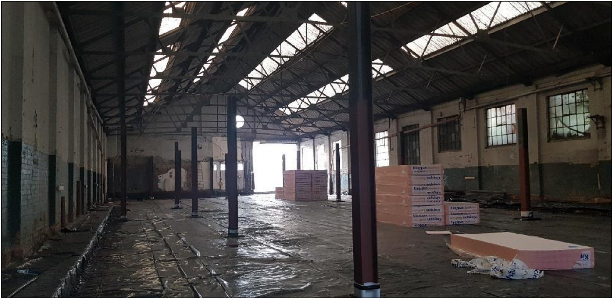
Photo 6: Looking south across the interior of the main section of B1.
