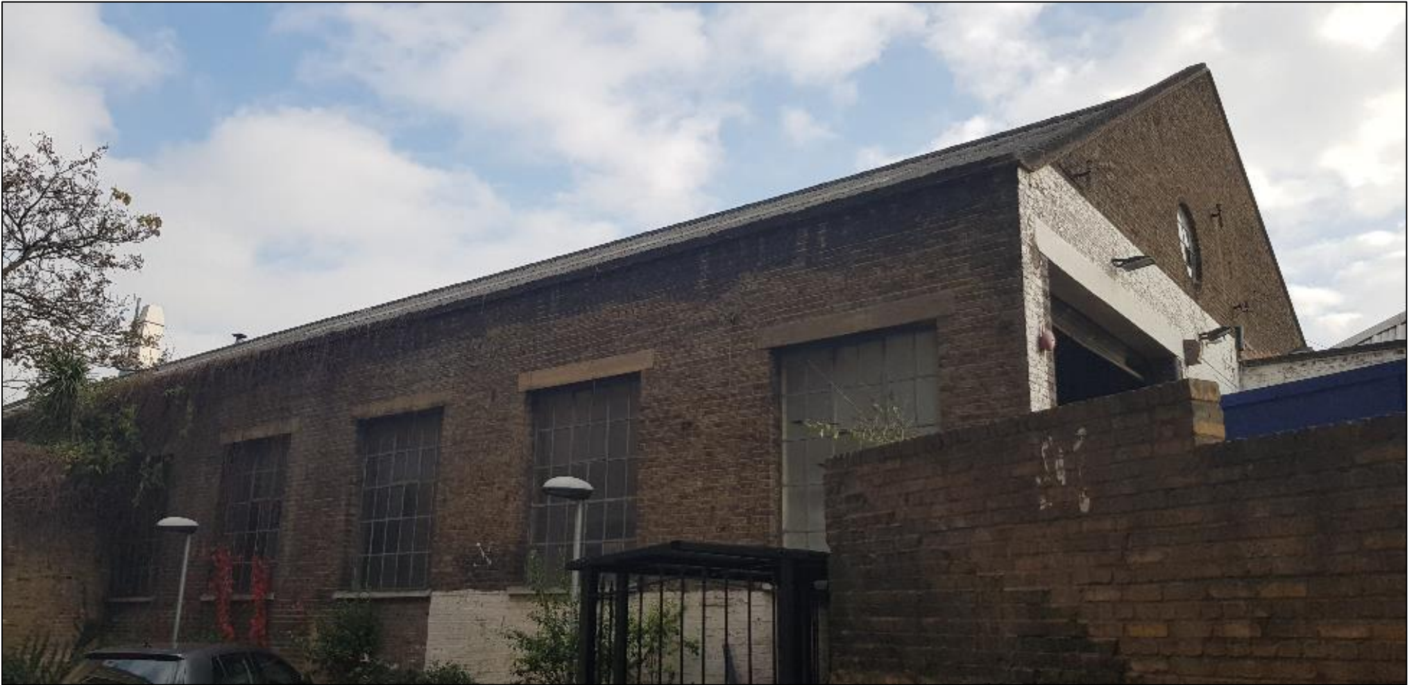
Photo 3: Western elevation of the main section of B1.
