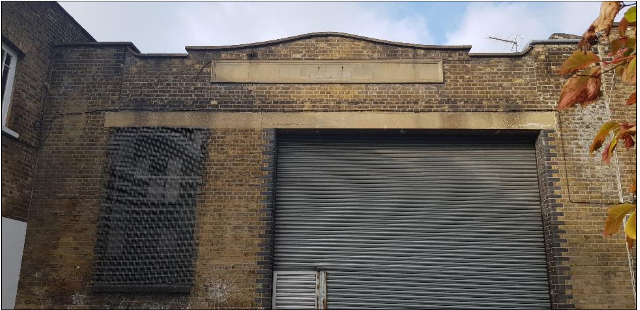
Photo 2: Eastern elevation of the main section of B1.
