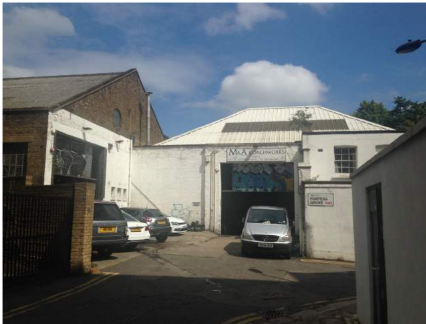
Figure 10: Entrance to the Site from Fortress Grove. The prominent corrugated metal roof largely detracts from the general quality of the Kentish Town Conservation Area.
