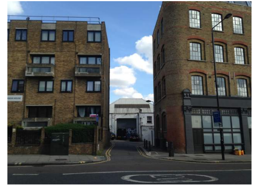
Figure 12: The Site as viewed from Fortress Road
