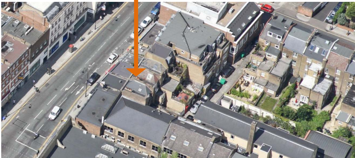
2 Aerial View of showing the rear of 162 Kentish Town Road
