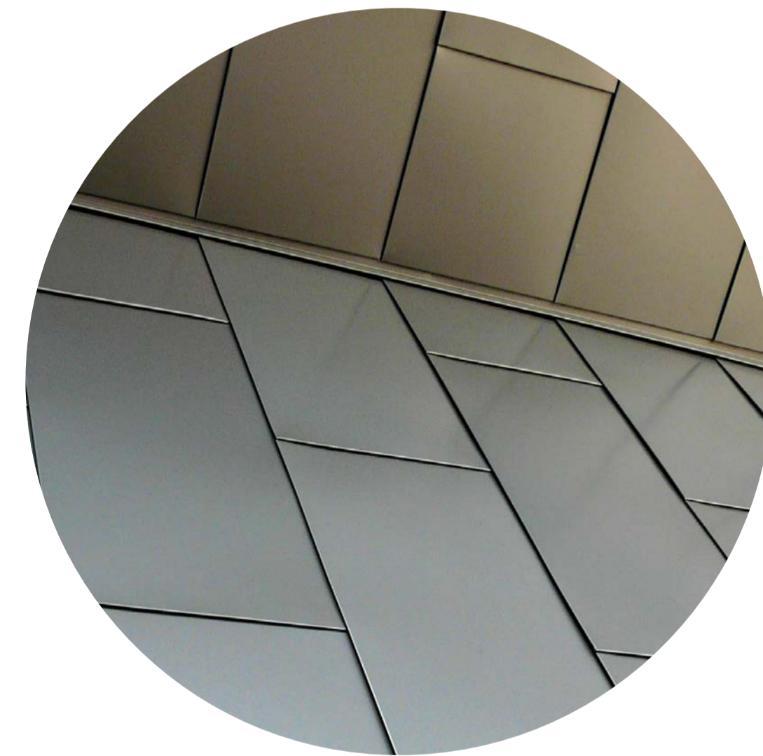
Zinc Cladding Location - Block A Undercroft Linings / Level 4 Cladding Manufacturer - VM Zinc or similar Product - Anthra Zinc
