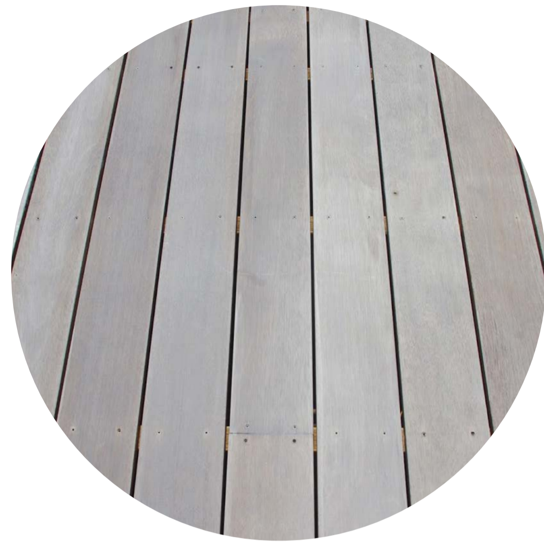
Timber Cladding and Decking Location - Block B Terraces Generally Natural Larch, finished with Osmo White Natural Woodstain or similar
