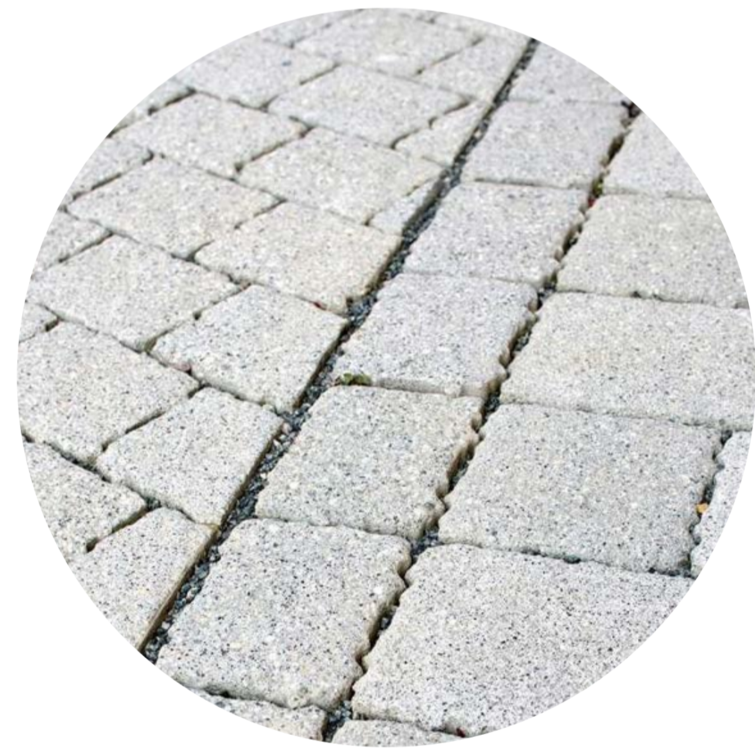
Light Grey Permeable Paving Location - Central Courtyard Manufacturer - Marshalls Product - Mistral Priora Colour - Silver Grey
