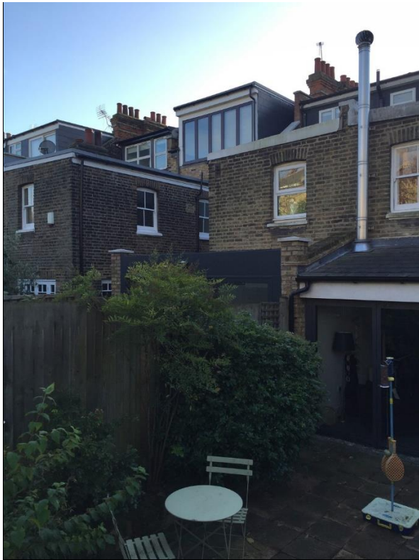
Photograph showing the variety of rear roof extensions surrounding the application site.
