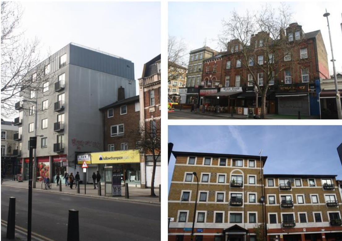
VARIETY IN SCALE, HEIGHT AND DESIGN OF NEIGHBOURING BUILDINGS (LEFT: 375 KILBURN HIGH ROAD UPPER RIGHT: 336-332 KILBURN HIGH ROAD LOWER RIGHT: SPRING COURT)
