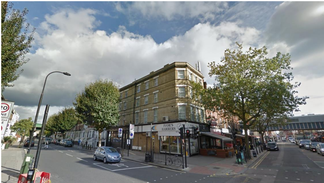
APPLICATION SITE VIEWED FROM JUNCTION
