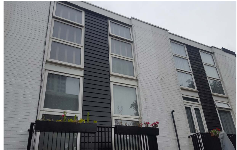
Rear view of No 4 Briary Close
