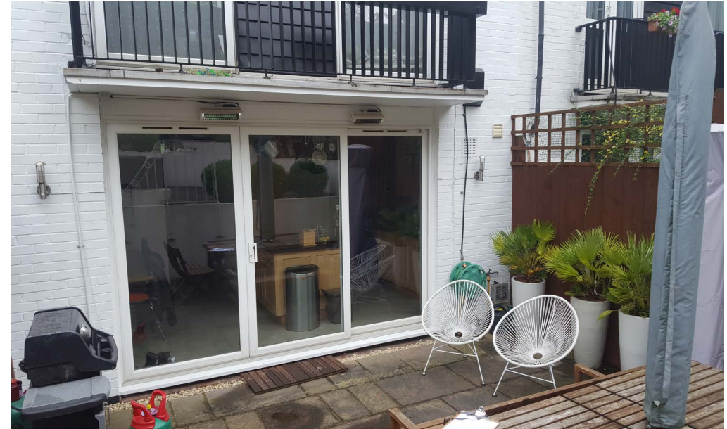
Rear view of No 4 Briary Close
