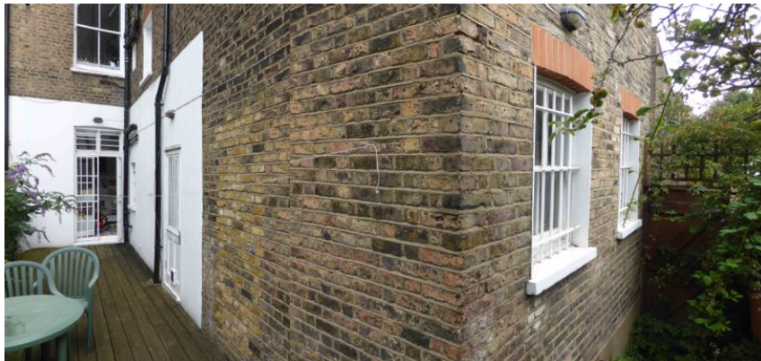
Fig 3 photograph of West garden elevation – rear windows to be extended to floor level (one converted to a door), render renewed and extended almost to corner.
