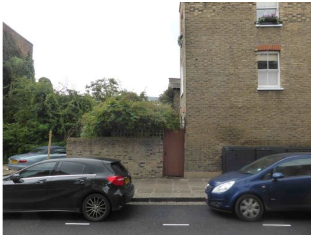
Fig.1 photograph of side of ground floor extension – arches to rear windows visible (no alteration proposed)
