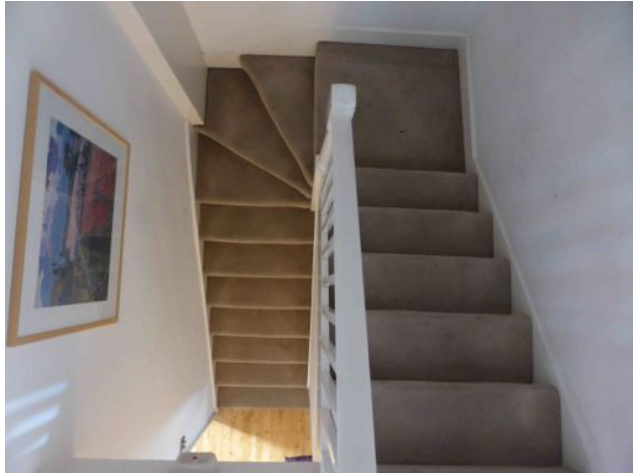
Fig 4 photograph of cranked stair- difficulty for mobility impaired use to visit living spaces currently located on first floor.
