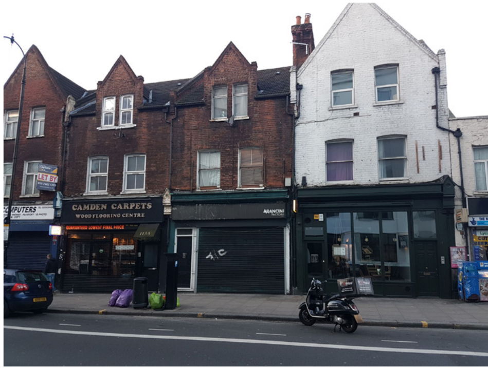
Existing brick façade to adjoining three storey properties
