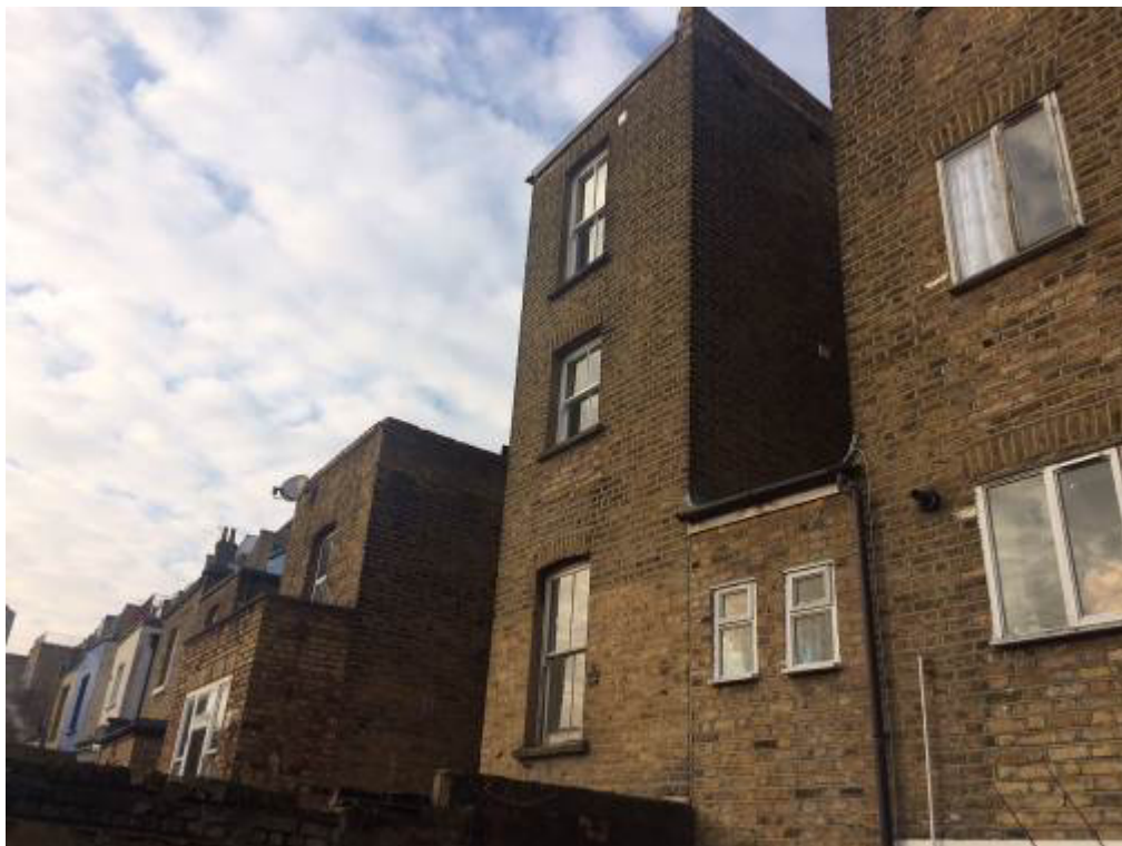
5. West side view of the rear of the terrace row
