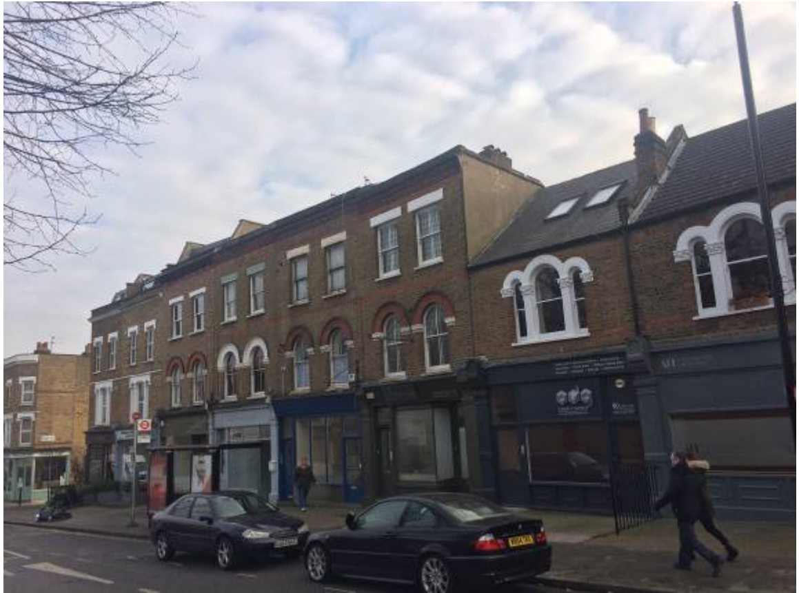
3 View to the east along Mill Lane
