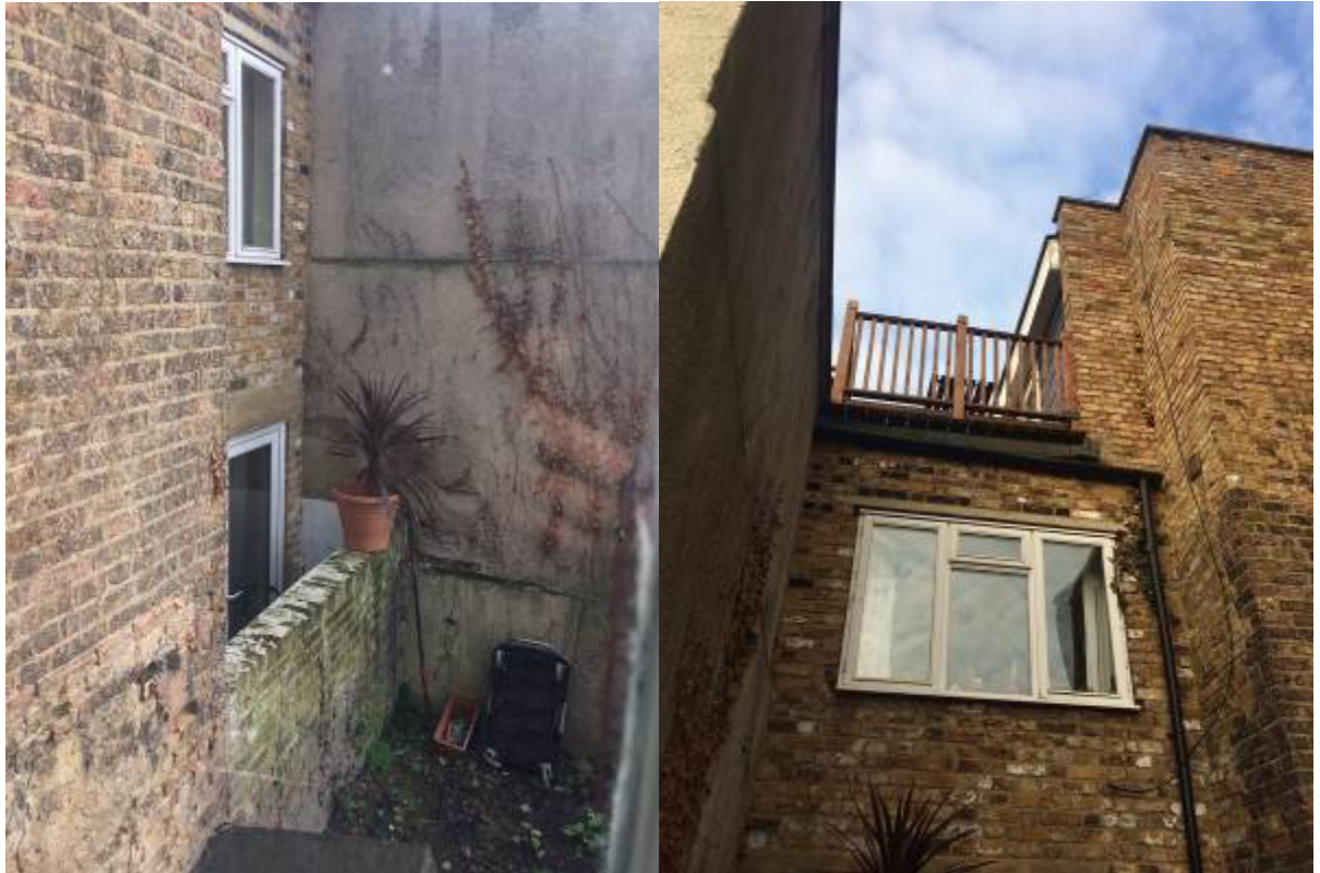
6. View towards the side/rear of No. 88 Mill Lane
