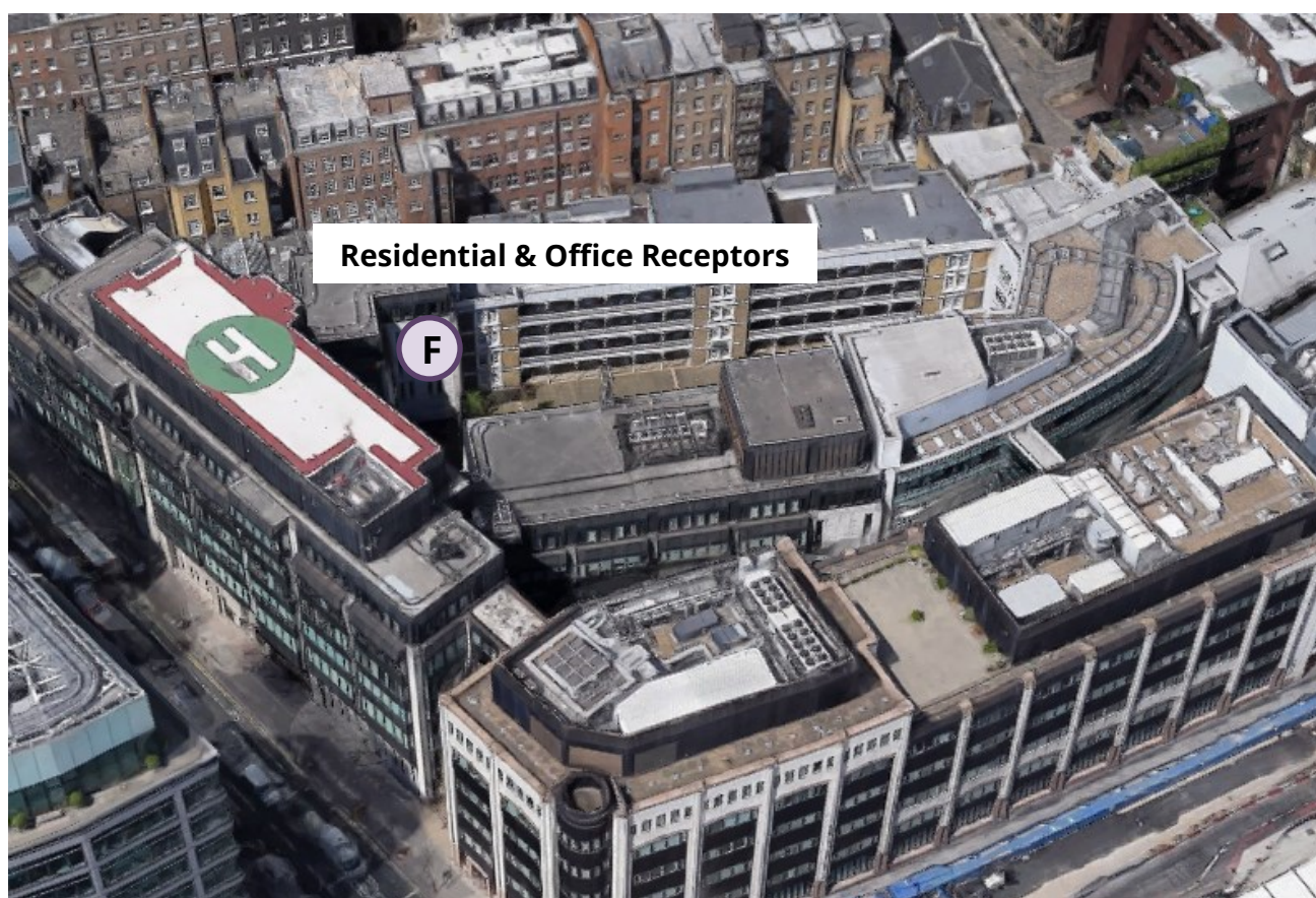
Figure 2.1: Site and Measurement Location
