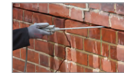
2. Clean out slots and flush with clean water and thoroughly soak the substrate within the slot
