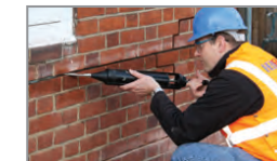
3. Using the Helifix Pointing Gun, inject a bead of HeliBond along the back of the slot
