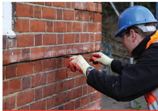
HeliBar is inserted into HeliBond grout within a cut slot
