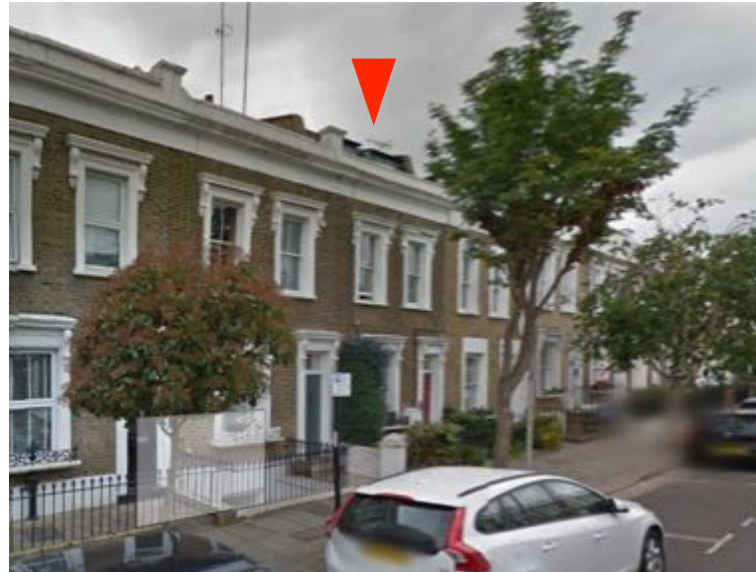
1. View of 8 Alma Street looking north
