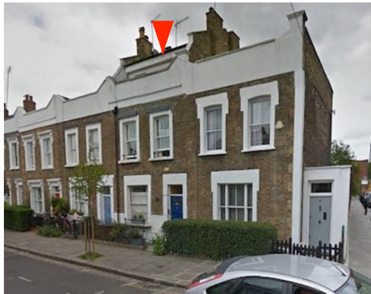
2. View of 21 Alma Street looking south
