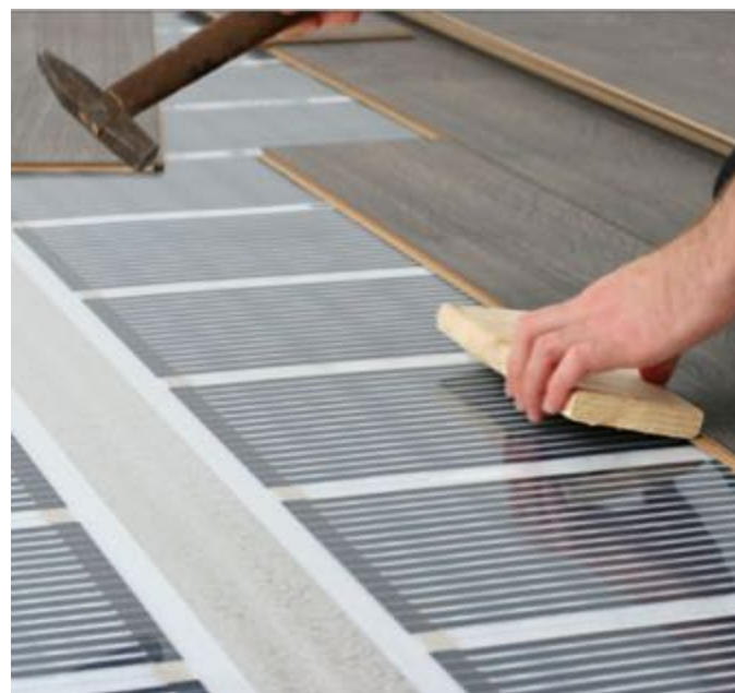
4. Underfloor heating installation - electric membrane low consumption
