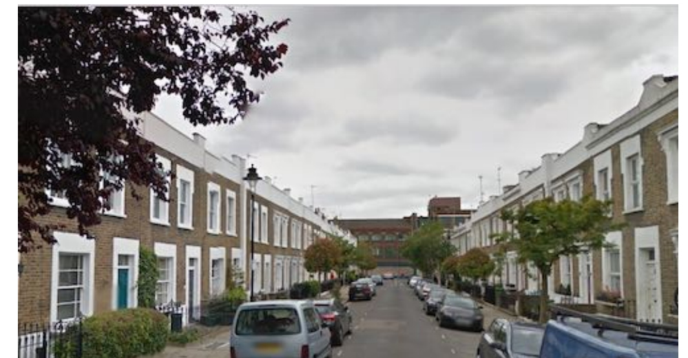
View of Alma Street looking south east
