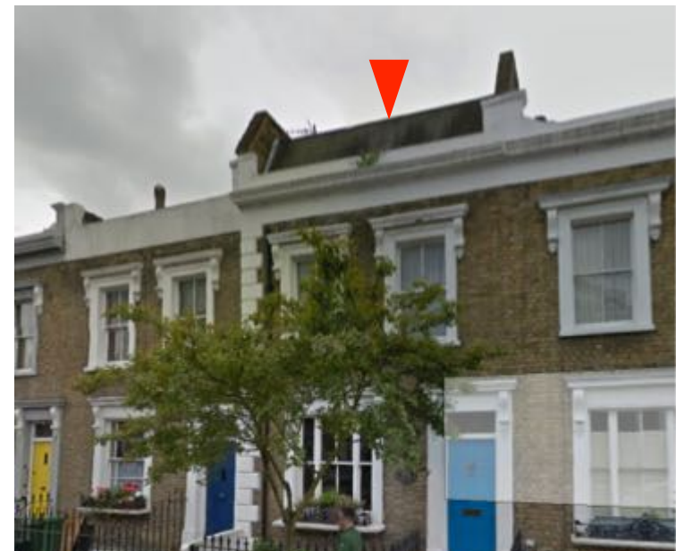
3. View of 51 Alma Street looking north
