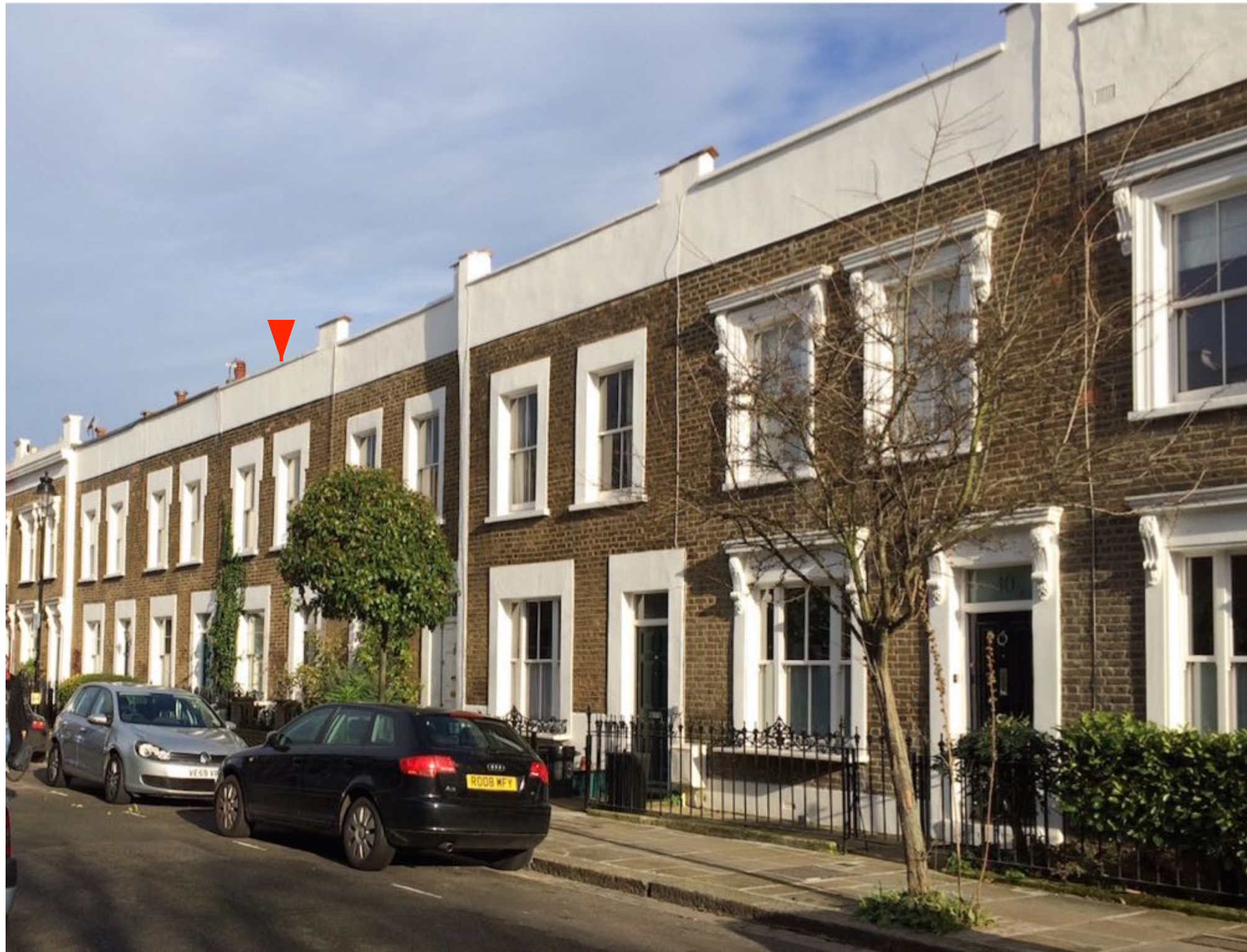
View of Alma Street seen from the south east (n.37 marked with an arrow)
