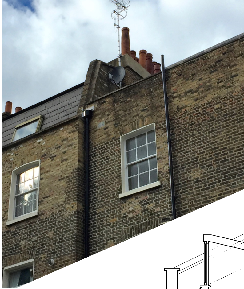
EXAMPLE OF IRS INSTALLATION - SATELLITE DISH (PAINTED BLACK), TV & RADIO AERIALS (at 33 FREDERICK STREET)
