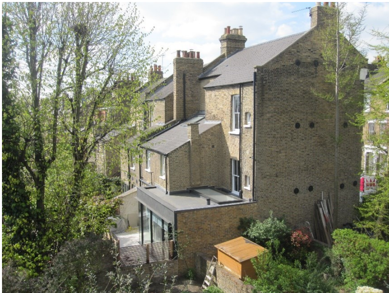
Rear extension at No. 56 Roderick Rd
