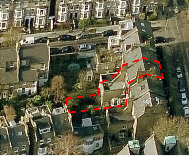
Aerial view of side elevation looking West
