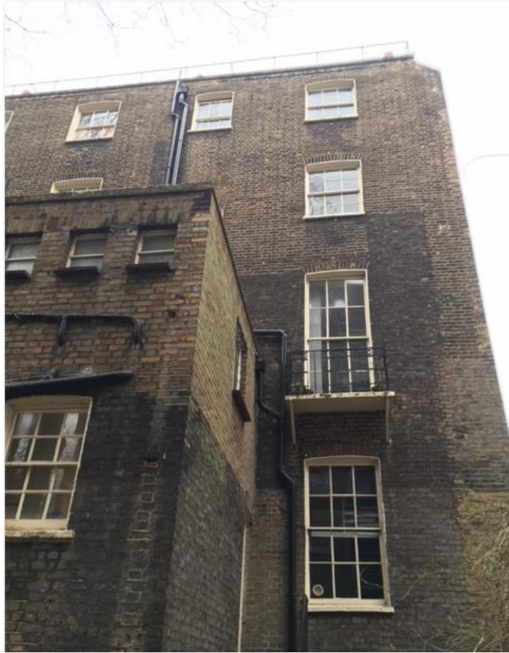
Photo 5: Rear elevation of no.32
