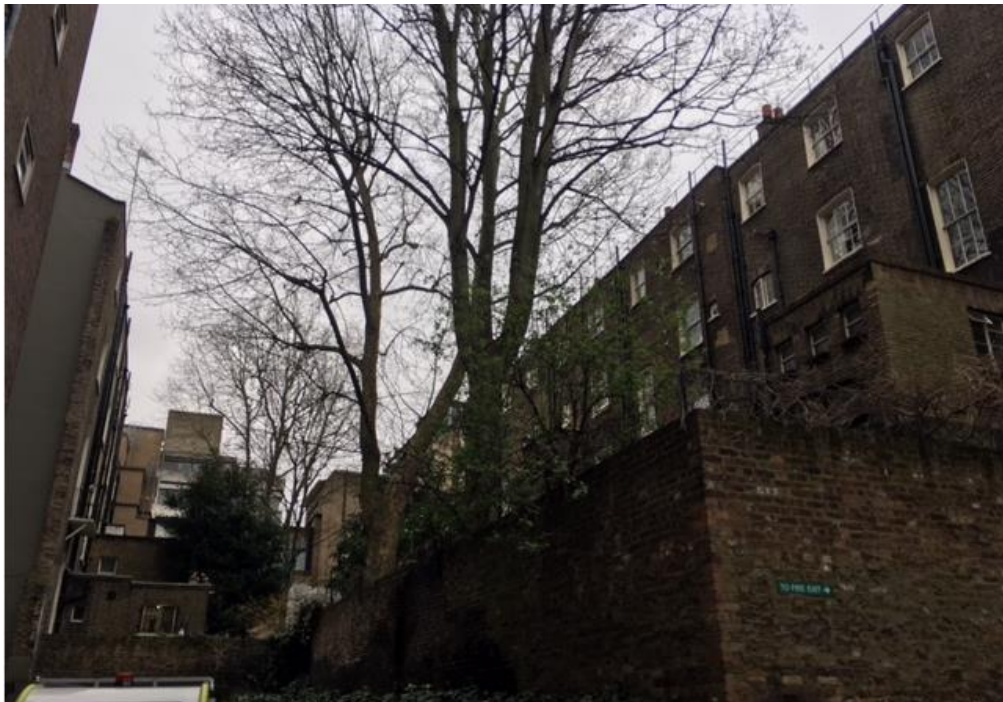
Photo 7: Looking south along the rear of the terrace
