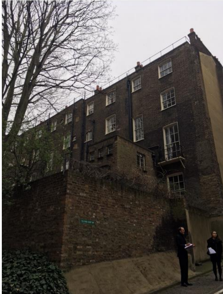
Photo 6: Rear elevation of no.32 and rest of terrace
