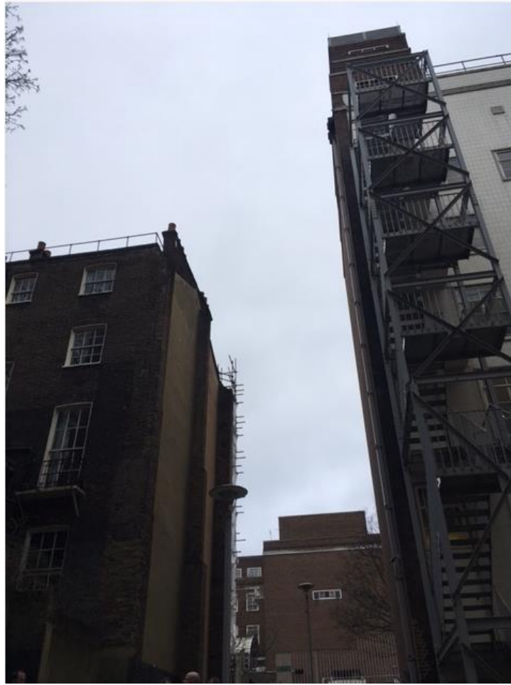
Photo 8: Looking west through the gap between no.32 and the Warburg Institute
