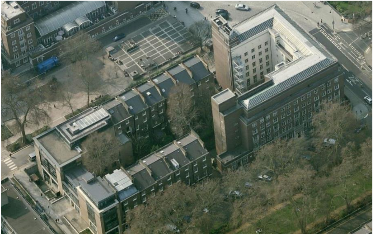
Photo 3: Aerial view looking west showing rear elevation
