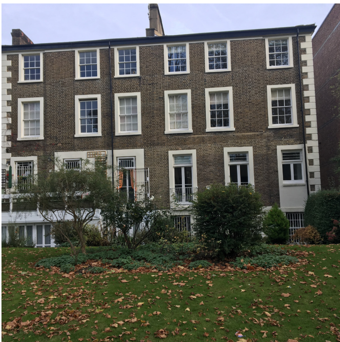
Rear elevation view of no. 45 & 43 Gloucester Avenue. Note the asymmetry caused by the existence of the rear extension at no. 45 but not at 43
