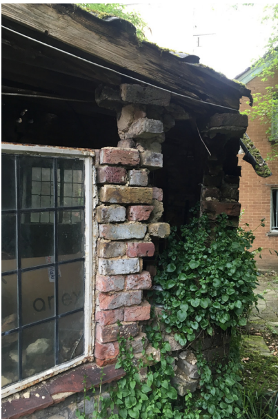
South-east view of existing external wall, showing large areas of missing bricks, cracks and bowing.
