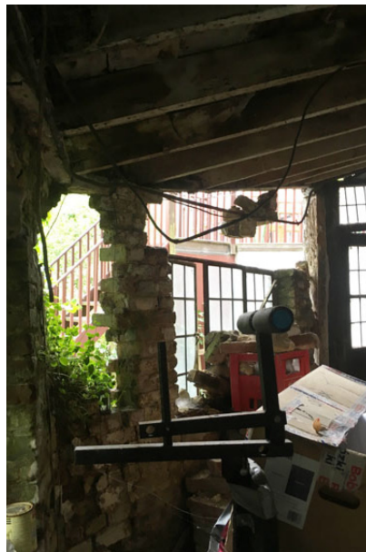
Internal view looking south, the existing roof supported by an insecure brick pier.
