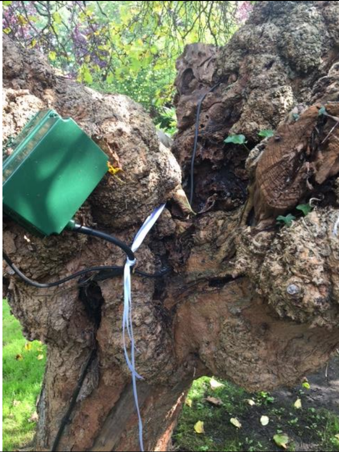
T3 - Trifurcation area partially collapsed in Mulberry.
