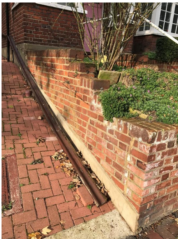
View 4 – Garden retaining wall
