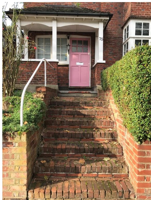
View 5 – Front entrance steps and porch
