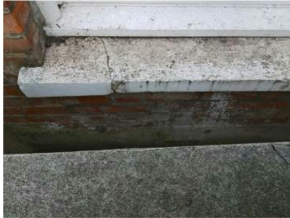
Fig 01 – Below front bay
