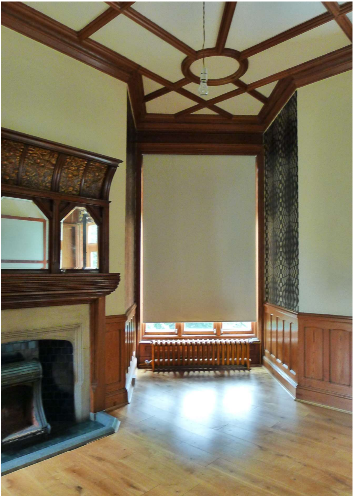
A2.3 View within the former Morning Room, proposed for conversion to a kitchen, showing the retained fireplace and modern engineered oak flooring.
