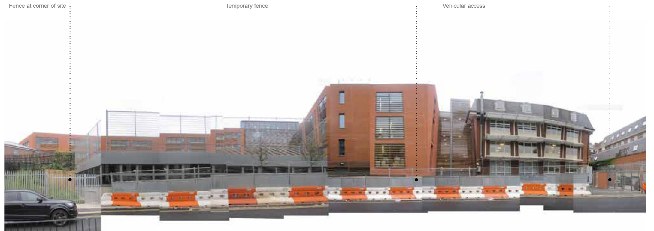
Panorama of existing street elevation
