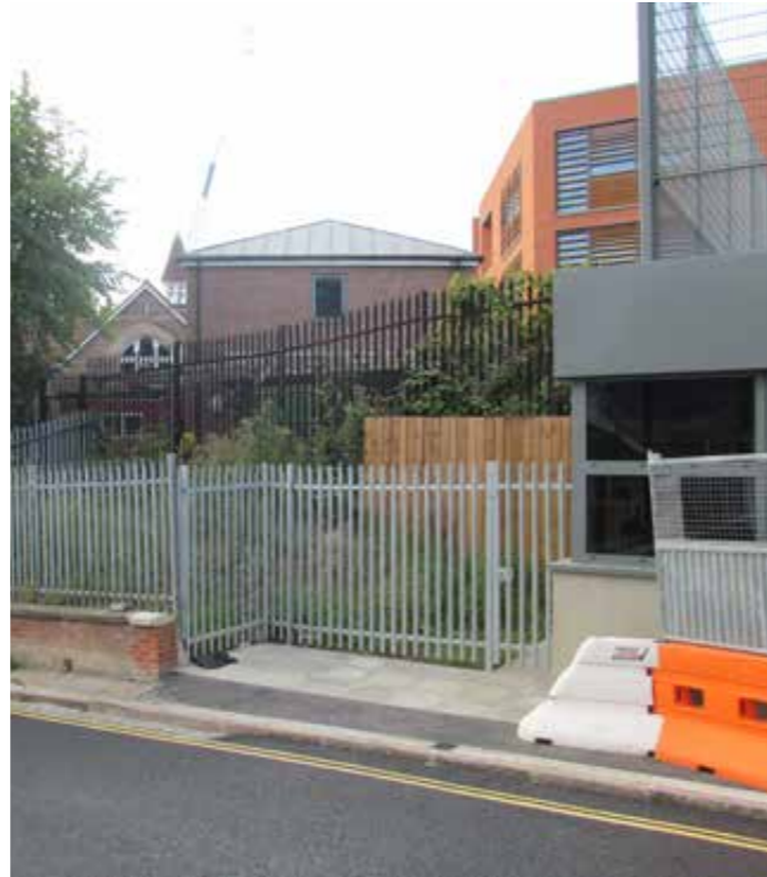
Fence at corner of site
