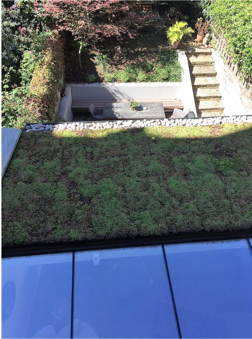
EXAMPLE OF SEDUM GREEN ROOF AT GLOUCESTER CRESCENT
