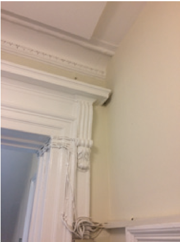
Original cornice in lobby broken by non-original partition
