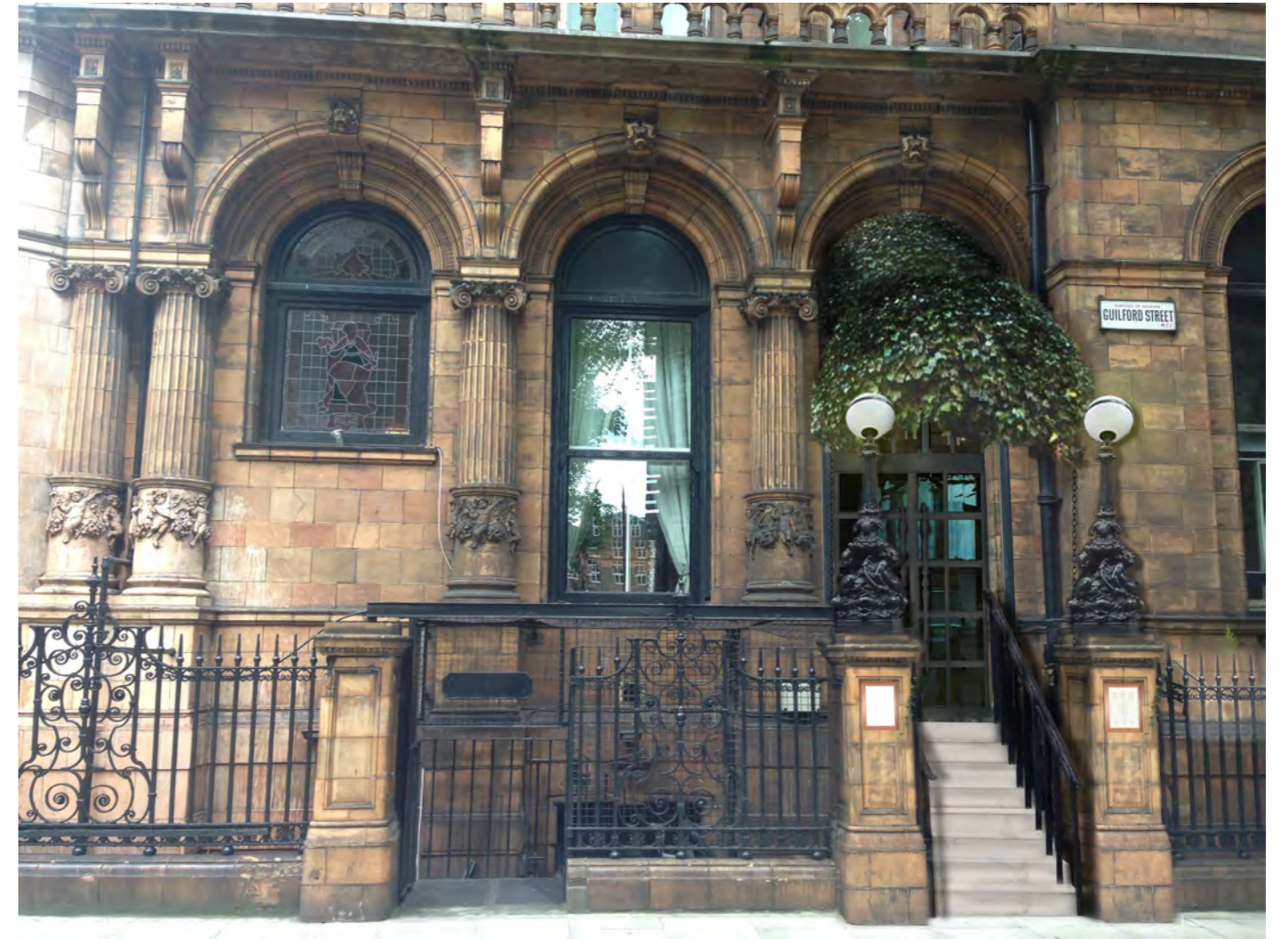
Figure 15: Indicative CGI of the projecting canopy and ivy cladding from Guildford Street
