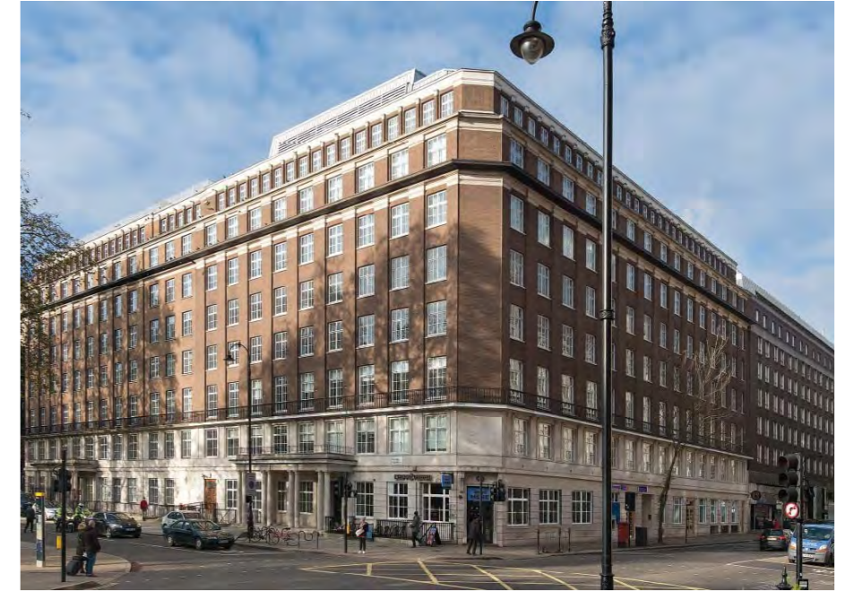
Figure 6: Russell Square House, Russell Square. Noted for being a positive building within the Sub Area 6: Bloomsbury Square/Russell Square/Tavistock Square conservation area (Source: http://russellsquarehouse.london/ )
