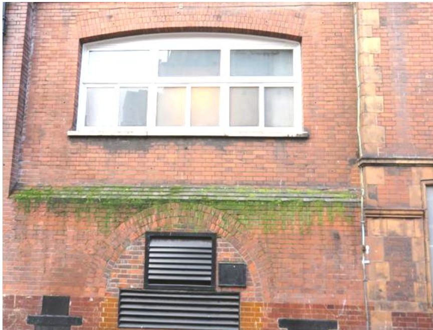
Figure 26: Evidence of moss and algae on Herbrand Street brick wall (Source: Peter Harrison Mark Goldman Design Consultants Ltd, External Façade Condition Survey covering; Herbrand Street, dated 12 February 2015).
