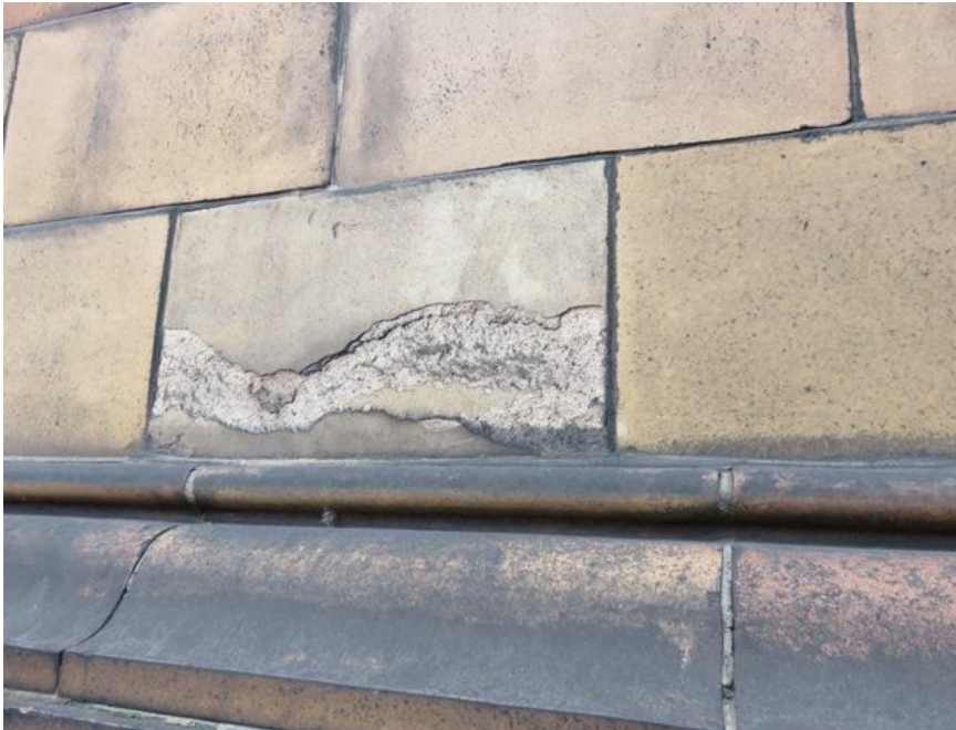
Figure 27: Areas of terracotta failure on Herbrand Street (Source: Peter Harrison Mark Goldman Design Consultants Ltd, External Façade Condition Survey covering; Herbrand Street, dated 12 February 2015).
