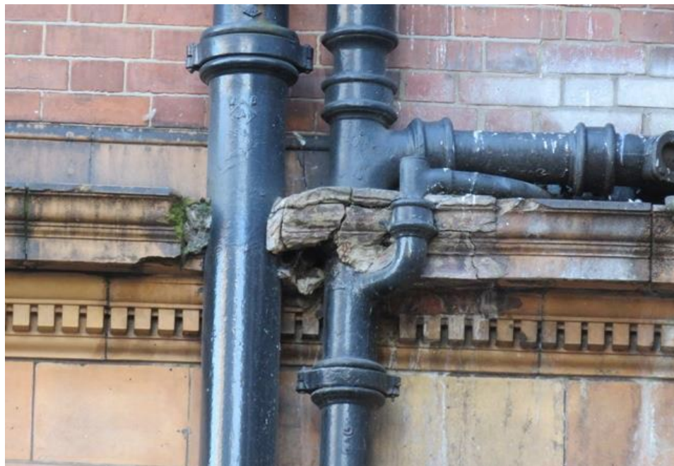
Figure 25: Pipework installed through terracotta dentilled cornice. (Source: Peter Harrison Mark Goldman Design Consultants Ltd, Russell Hotel: External façade Condition Survey covering; Russell Square, Bernard Street, Guildford Street, dated 10 February 2015).
