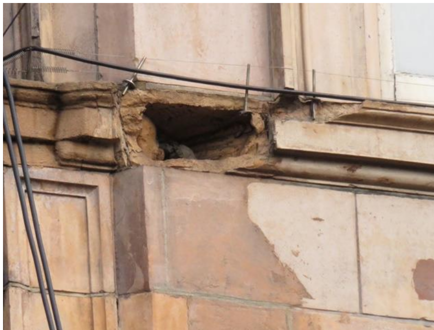
Figure 22: Failure of terracotta requiring replacement. (Source: Peter Harrison Mark Goldman Design Consultants Ltd, Russell Hotel: External Façade Condition Survey covering; Russell Square, Bernard Street, Guildford Street, dated 10 February 2015).
