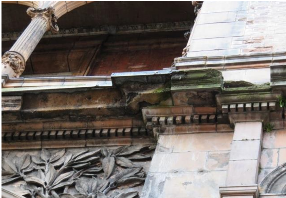
Figure 24: Damage to the terracotta cornice caused by water leakage over a long period of time (Source: Peter Harrison Mark Goldman Design Consultants Ltd, Russell Hotel: External façade Condition Survey covering; Russell Square, Bernard Street, Guildford Street, dated 10 February 2015).
