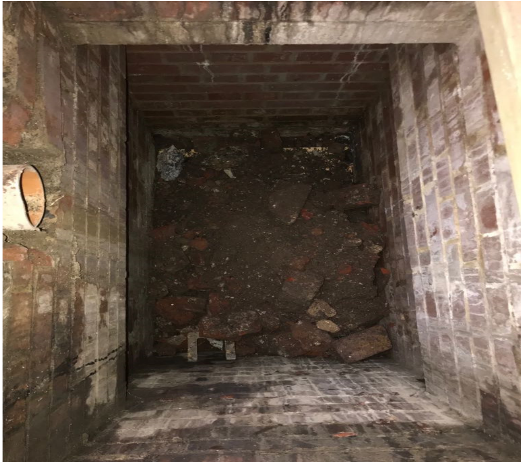
10-11 Kings Mews- existing manhole filled to prevent ingress of rodents
