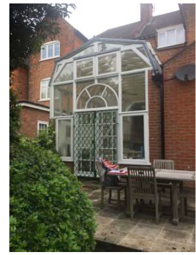
PHOTOGRAPH OF EXISTING CONSERVATORY
