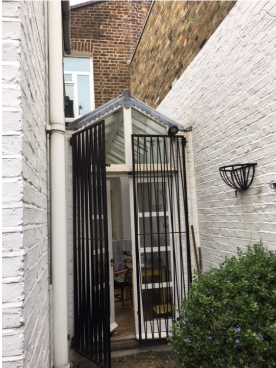
Existing rear infill extension
