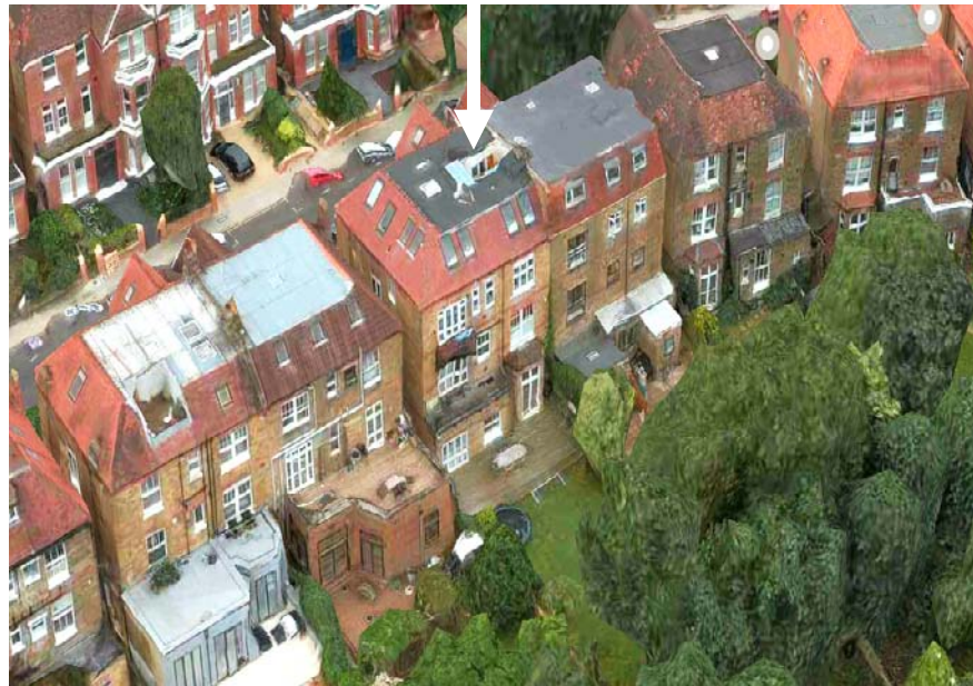
4. Aerial View showing rear of No. 60 Canfield Gardens
