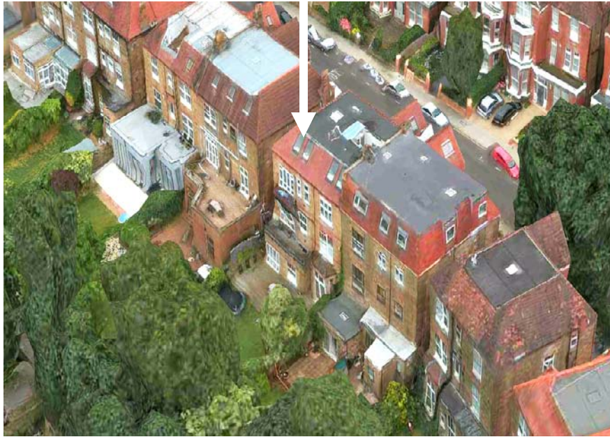
3. Aerial View showing rear of No. 60 Canfield Gardens
