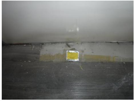
Material Comments: A sample of lino to floor (green) was removed for laboratory bulk sampling analysis from the retail at ground floor level. Note -Below screed.
