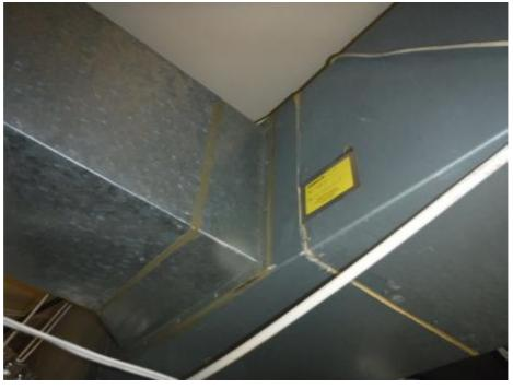
Material Comments: A sample of mastic to ducting was removed for laboratory bulk sampling analysis from the office area ceiling void at basement level.
