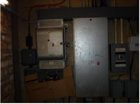
Material Comments: A photographic reference of electics within the electrical cupboard at basement level, strongly presumed to contain asbestos i.e flash pads, ropes, gaskets etc. Note - Electrics were live at time of survey.
