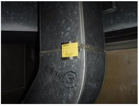
Material Comments: A sample of mastic to ducting was removed for laboratory bulk sampling analysis from the a/c room at mezzanine level. NOTE - Mastic to ducting was noted throughout.
