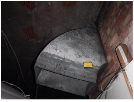
Material Comments: A sample of residue to ducting was removed for laboratory bulk sampling analysis from the retail ceiling void at ground floor
