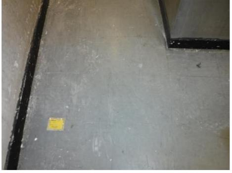
Material Comments: A sample of floor tile was removed for laboratory bulk sampling analysis from the corridor at ground floor level.
