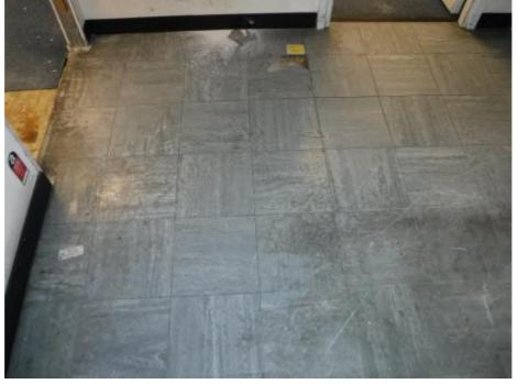
Material Comments: A sample of floor tile (dark grey) was removed for laboratory bulk sampling analysis from the hall at basement level.
