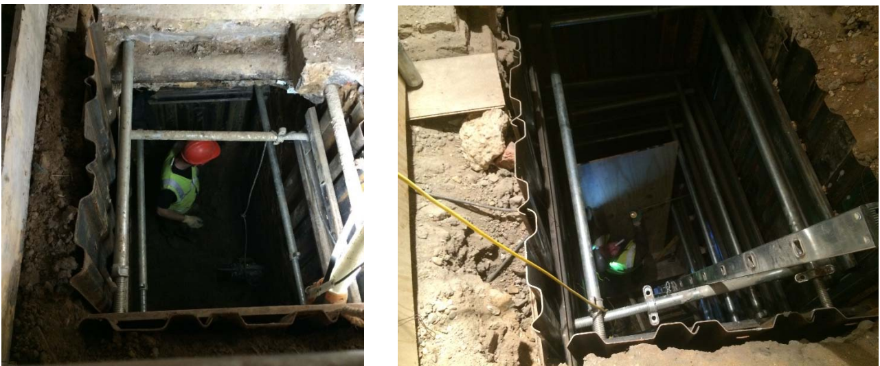
Figure 16 Examples of excavations of pins
