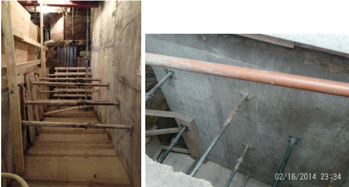
Figure 17 Examples of completed walls and back propping to central soil mass
