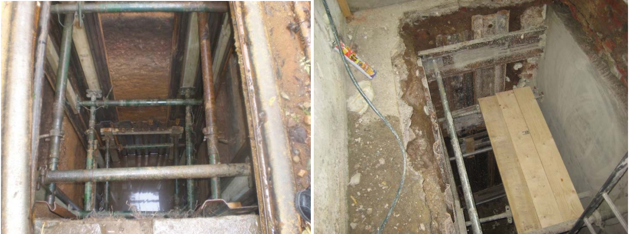
Figure 15 Propping examples
