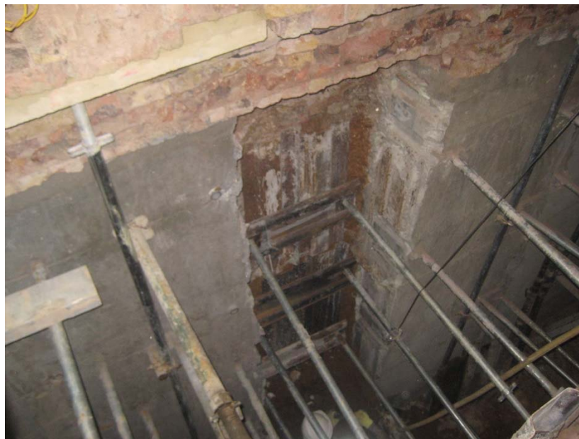
Figure 18 Example of trench sheet back propping
