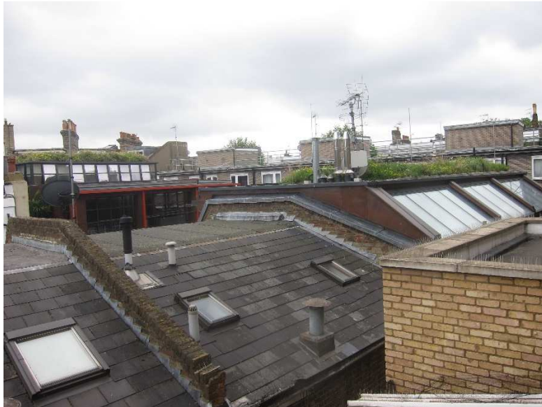
Photo 2-View from Application Site of existing development at rear
