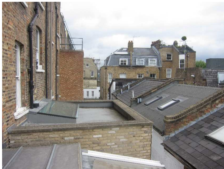
Photo 1- Rear View of Terrace with existing extensions shown
