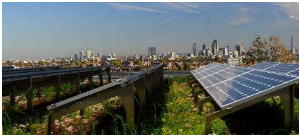
Figure 13. Indicative PV / green roof arrangement
