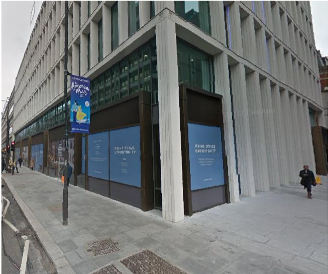
Photo 1- Retail Unit Corner of Bedford Avenue and Tottenham Court Road
