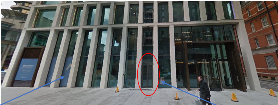
Photo 2- Bedford Avenue Elevation
