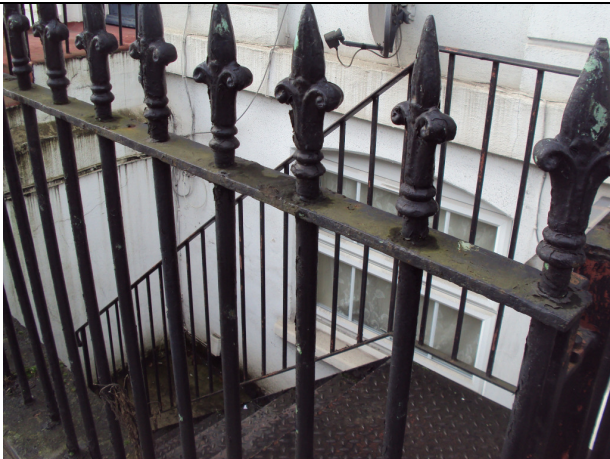
Figure 3 Railings to Lightwell
