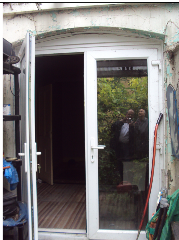
Figure 6 French Doors to Lower Ground Floor
