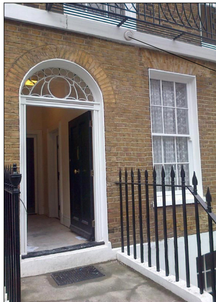
PROPOSED ELEVATION WITH EXISTING CABLING AND SECURITY LIGHT REMOVED
