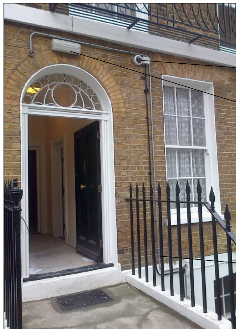
EXISTING ELEVATION WITH CCTV CAMERA AND CABLING
