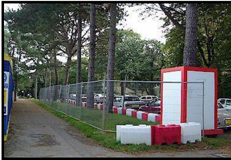
Pic 1: Example tree protection box.
