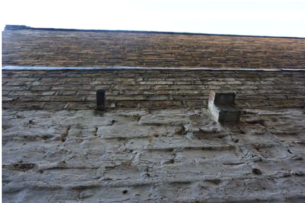
Flank wall showing flashing and old corbels
