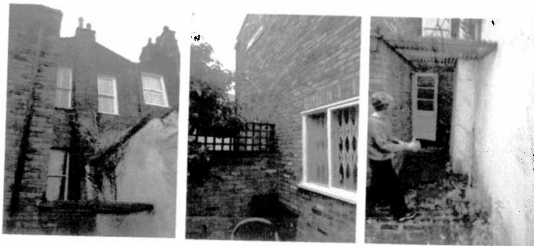
Existing photographs of the rear of the house
