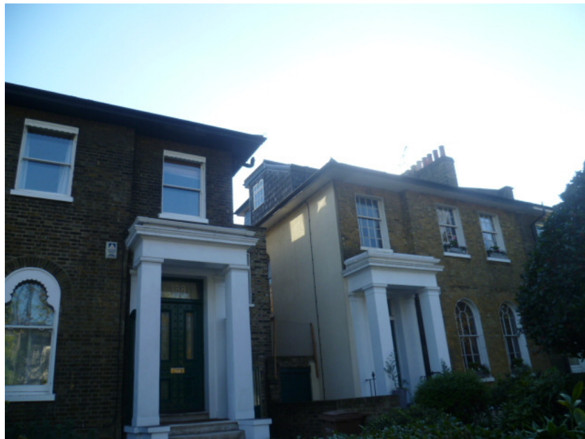
Photo No3 – View taken at street / pavement level of property No188
