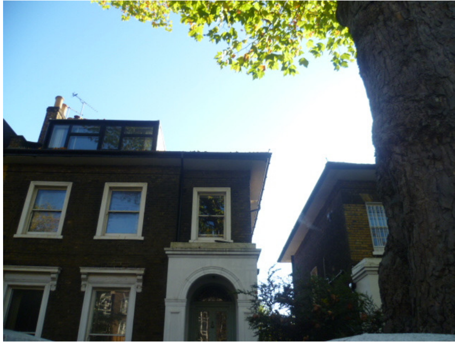
Photo No2 – View taken at street / pavement level next to the tree
