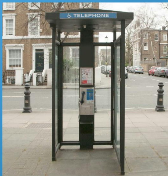
Front of the kiosk as seen from the pavement side showing open covered kiosk and accessible payphone
