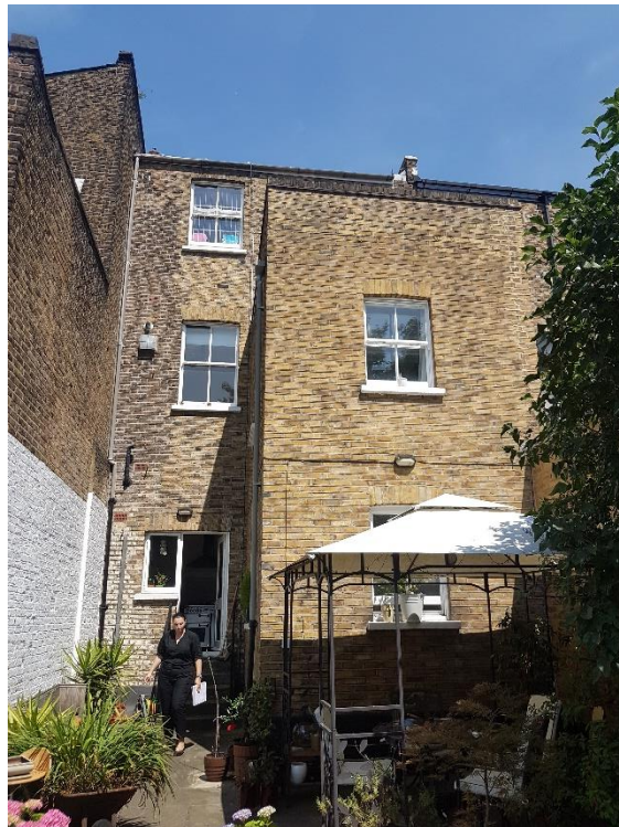
Rear elevation of the above addressed property at the ground floor
