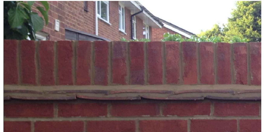
Photo of Brick on edge detail
