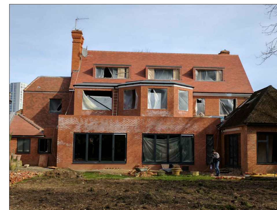
Photo of no 28 Harley Road First floor As Built
