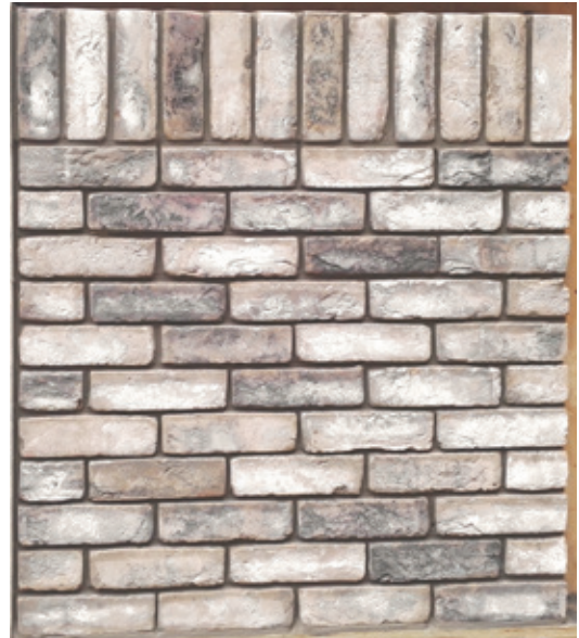
Photo of mock-up on site. Taken on 27.09.17
